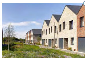
St. Chad's te Tilbury Essex Bell Phillips Architects
