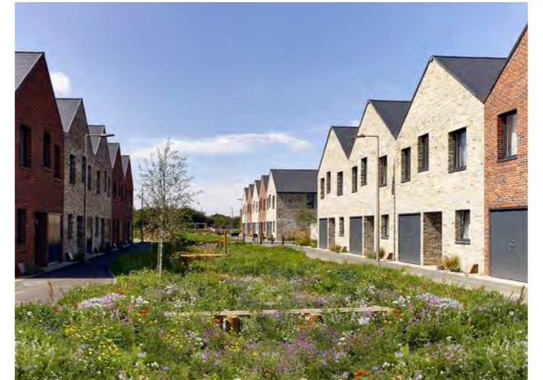
St. Chad's te Tilbury Essex Bell Phillips Architects
